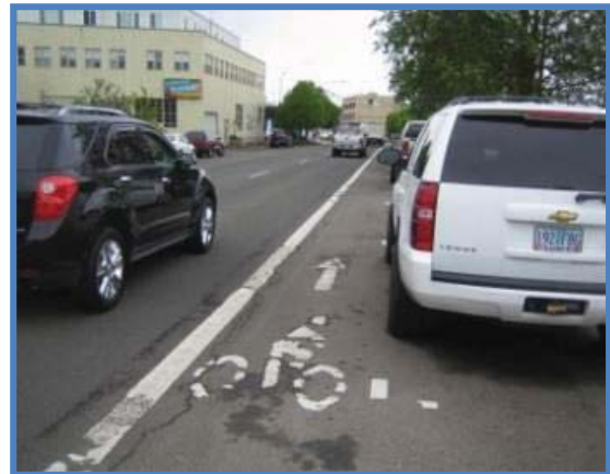
Narrow Bike Lanes on Marine Drive adjacent to parked vehicles
