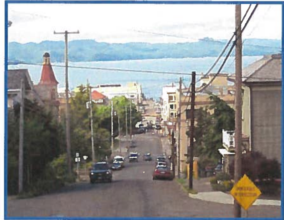
View from the Astoria hillside on 8 th Street
