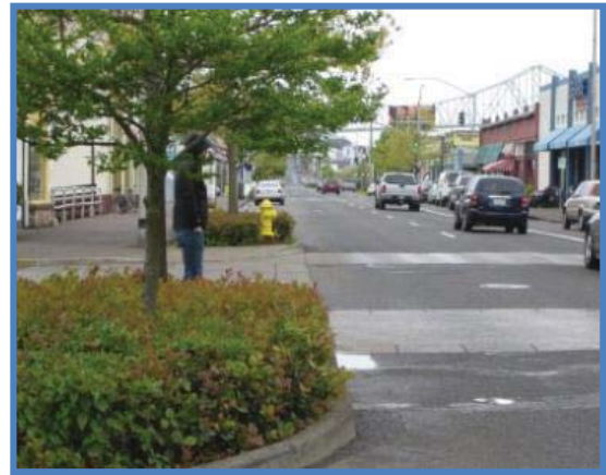
Curb extension on Marine Drive with vegetation obstructing the drivers view of the pedestrian
