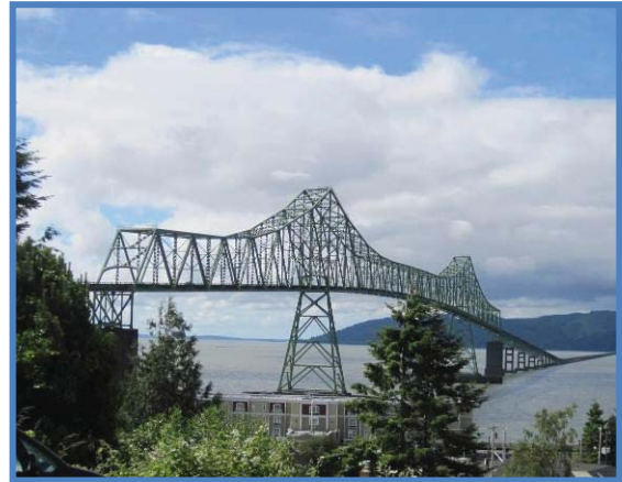
View of the Astoria-Megler Bridge from the City
