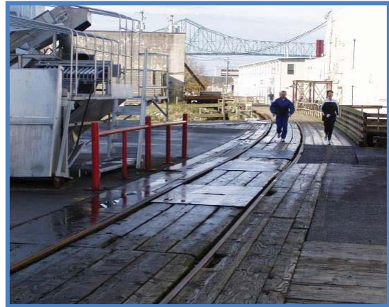
Wide gaps on the surface may be a safety concern for cyclists
