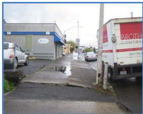
Sunken sidewalk on Marine Drive between 9 th and 10 th Streets downtown
