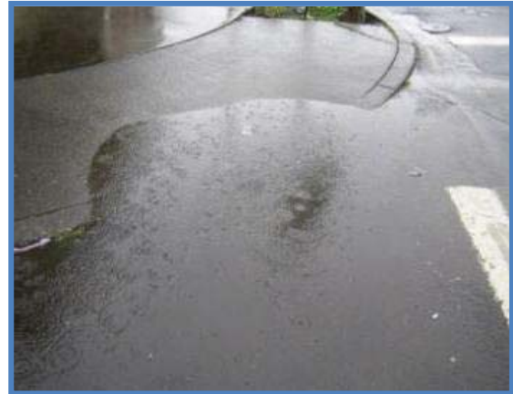
Drainage issues at a curb ramp downtown
