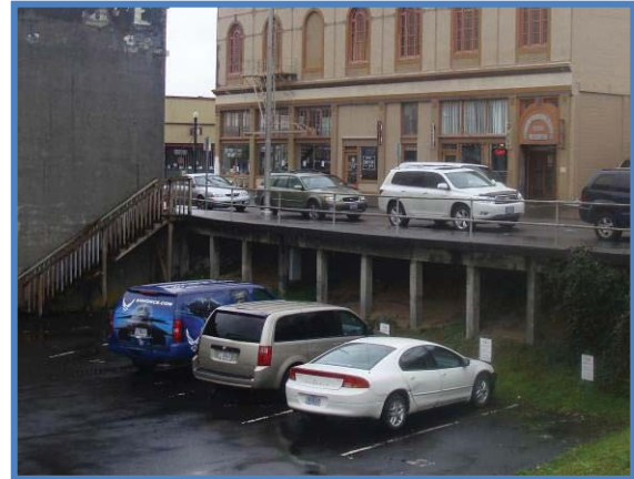
Exposed Chair-wall System at 10 th and Duane
