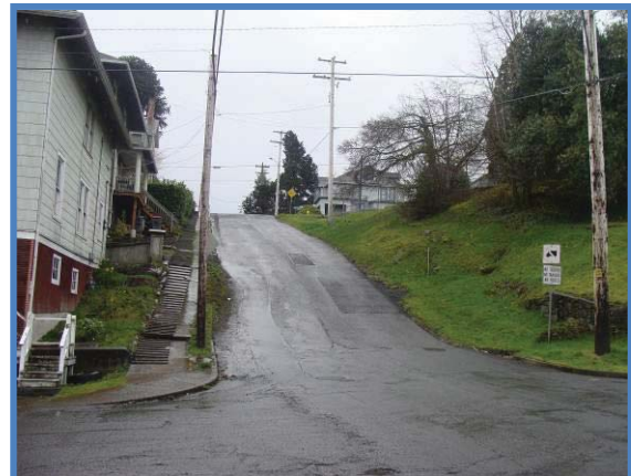
Steep hill with stairs in place of a sidewalk on 8 th Street
